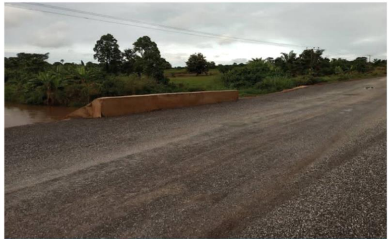
PROJECT DESCRIPTION: CONSTRUCTION OF ATONSUAGYA ROAD DIGITAL ADDRESS: AM-2553-2368
