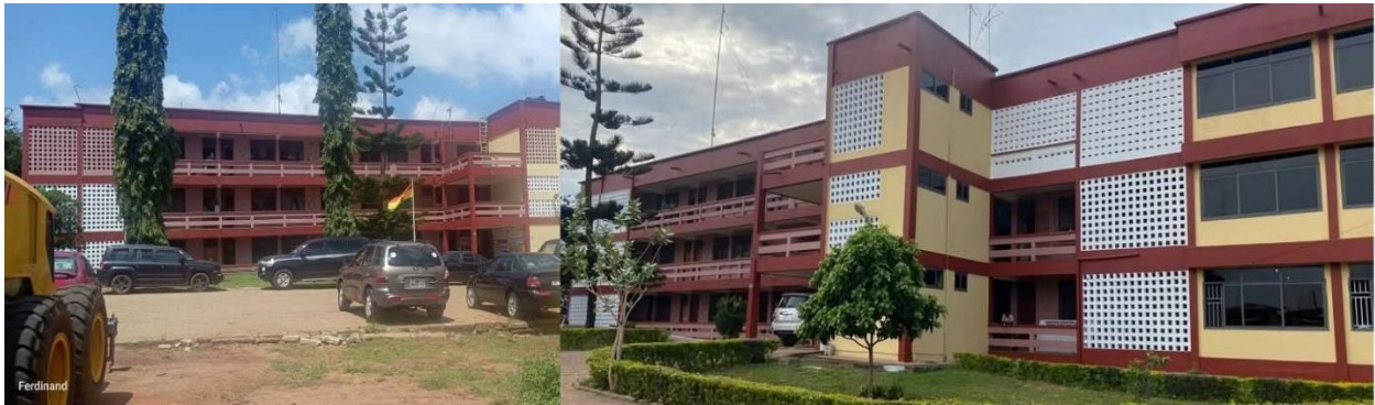
Renovated Assembly's Administration Office
