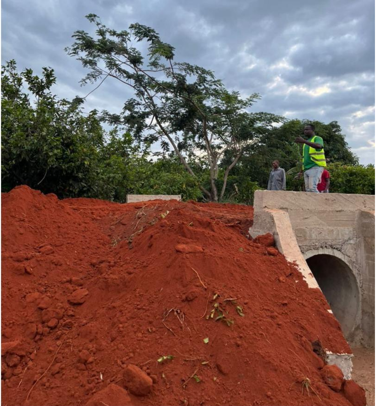
Completed Bridge linking Timber Nkwanta and Hiamankyene
