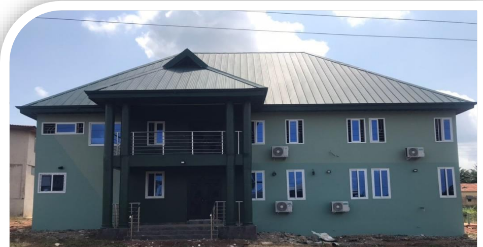
PROJECT DESCRIPTION: IMMIGRATION OFFICE LOCATION: MAMPONG SOURCE OF FUNDING: MR. MARFO AMPONSAH AKA AGYA WIASE DIGITAL ADDRESS: AM-0020-1172
